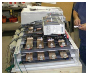
Insultemp® used on medium voltage electrical bus bar application to replace insulative rubber shrink boots. This presented a 70% cost reduction in materials
